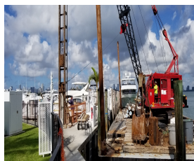
Pile Driving on E-Dock
